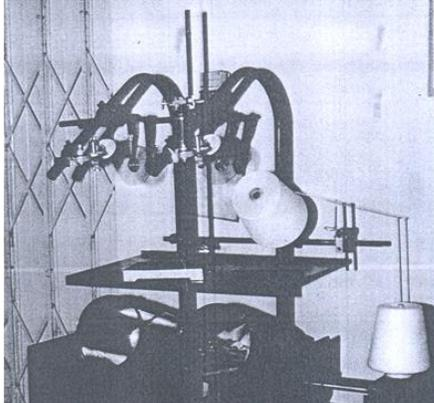
Fig. 1. High-speed pirn winding machine
