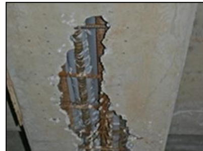
Figure 1 Concrete Honeycomb
